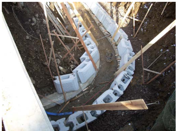
R = 1.0m、R = 3.0m敷設
