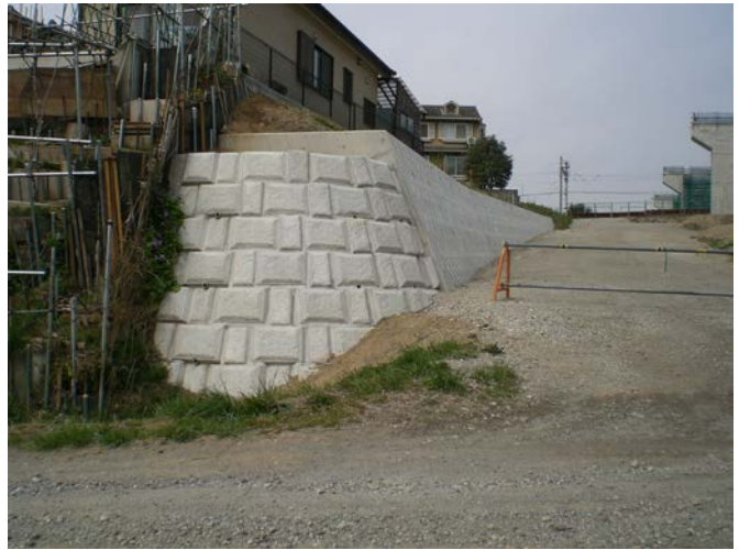
R = 1.8m 施工
